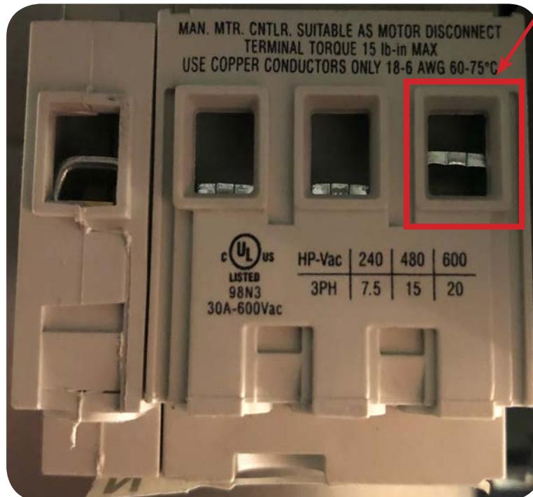
**IMPORTANT:** ensure wires are secure in the terminal.
